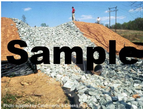
Photo 1 – Rock-lined sediment basin spillway with line outlet
