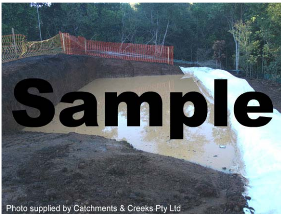
Photo 5 – Recessing the basin into the ground allows the natural ground level to become the spillway
