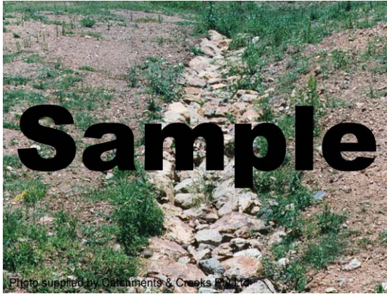
Photo 3 – An example of the rock-lining being correctly recessed into the topography
