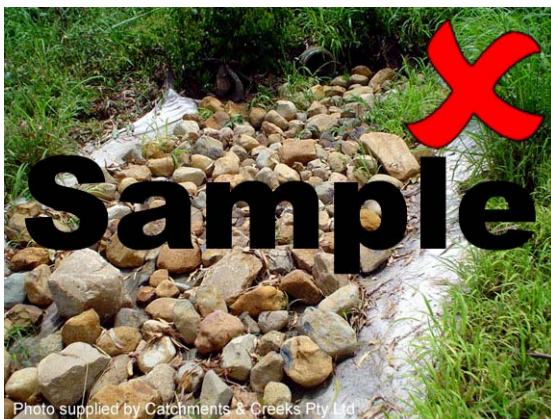
Photo 7 – Rounded rock can be significantly less stable than angular, fractured rock, especially when placed on steep slopes
