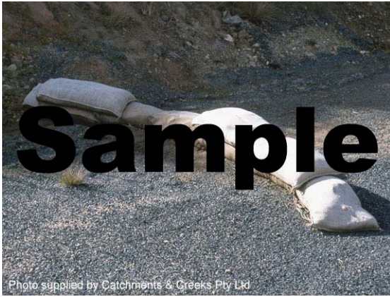
Photo 3 – Sandbag check dam
