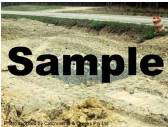
Photo 1 – Rock & aggregate drop inlet at road intersection
