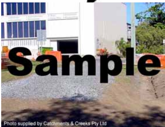
Photo 7 – Drain down-slope of rock pad directing sediment-laden runoff to a nearby sediment trap.
