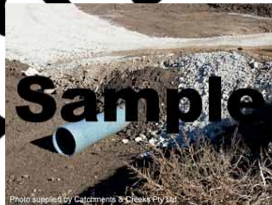
Photo 6 – Passing site runoff under a rock pad
