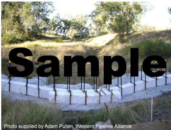
Photo 1 – Modular sediment trap
