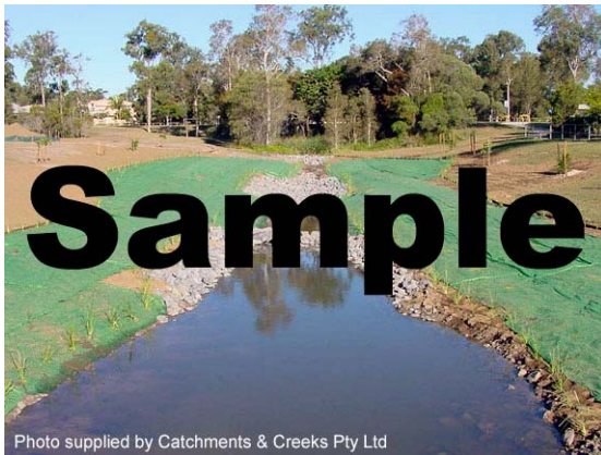
Photo 1 – Erosion control blankets installed during channel restoration
