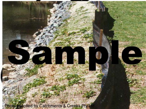
Photo 2 – Jute mesh scour protection on the upper bank and lower rock protection
