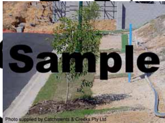
Photo 6 – Lateral strips of turf used to reduce the risk of rilling along the up-slope edge of the grassed filter strip
