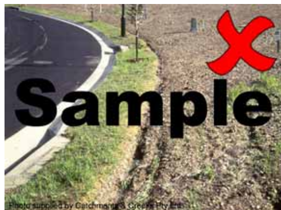
Photo 8 – Example of rilling caused by surface runoff being diverted along the up-slope edge of the turf
