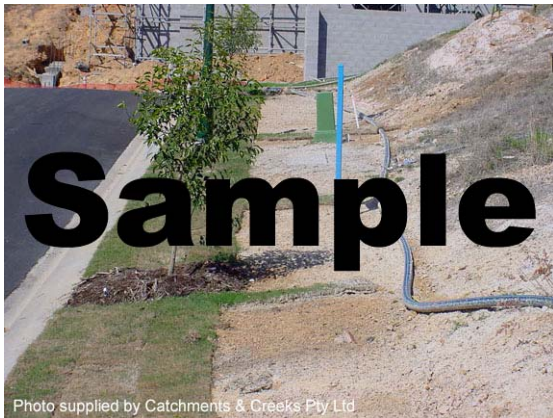
Photo 5 – Lateral inflows can reduce the risk of flow diversion along up-slope edge of turf
