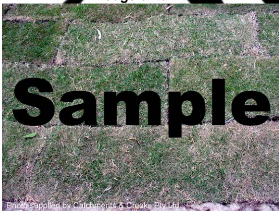
Photo 7 – Placement of turf in a “stretcher bond” form to reduce the risk of rill erosion occurring between individual strips of turf (flow is from top to bottom of photo)
