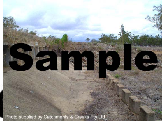
Photo 8 – Note use of impact blocks to stabilize the location of the hydraulic jump
