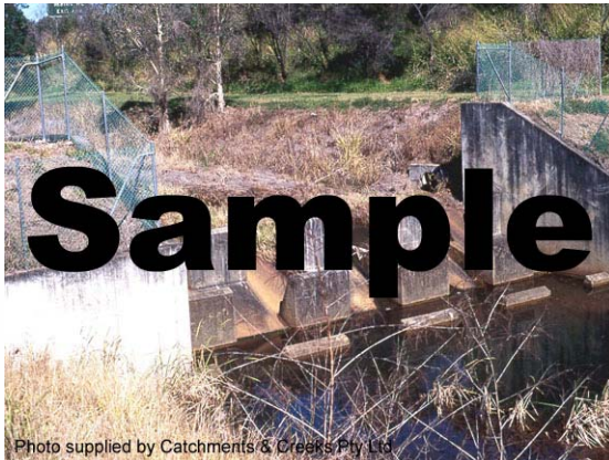
Photo 11 – Baffled spillway
