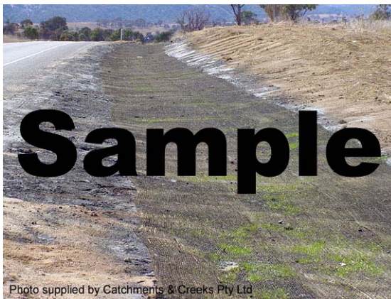
Photo 1 – Temporary jute mesh with emerging grass
