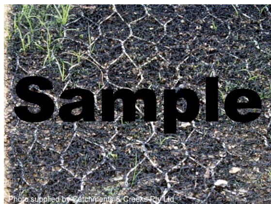
Photo 13 – Mat with additional mat reinforcing supplied by the wire mesh
