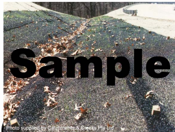
Photo 2 – Permanent, synthetic reinforced erosion control mat
