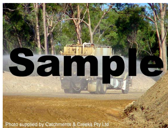
Photo 2 – Dust control using a water truck
