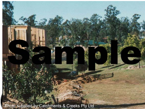
Photo 11 – Flow diversion bank up-slope of a building site – the bank also acts as a topsoil stockpile
