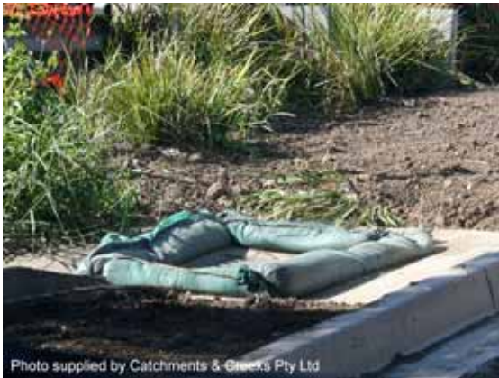
Photo 13 – Sandbags (filter sock)
