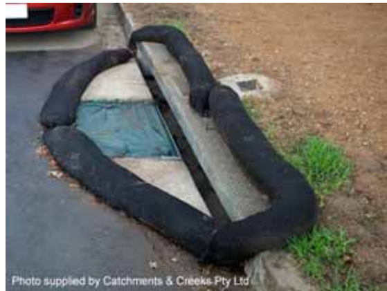
Photo 4 – Compost-filled filter sock
