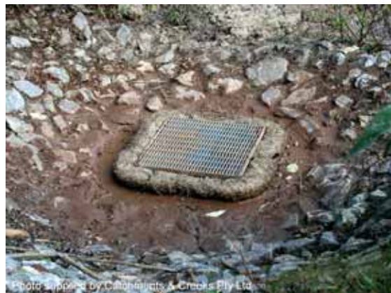
Photo 8 – Filter sock drop inlet protection
