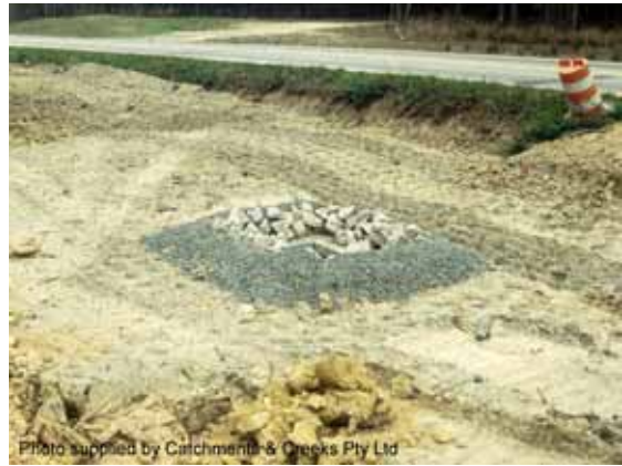
Photo 12 – Rock & aggregate system
