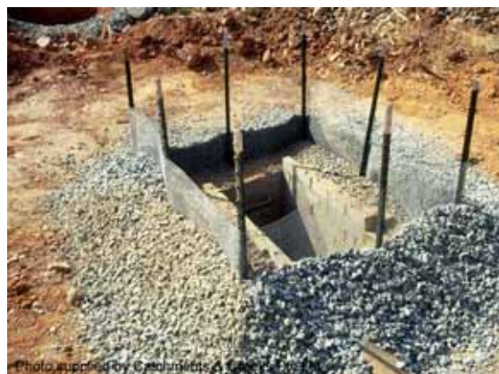
Photo 10 – Mesh & aggregate system
