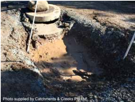
Photo 5 – Excavated drop inlet protection
