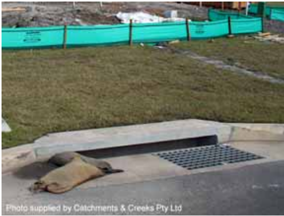
Photo 11 – On-grade kerb inlet control
