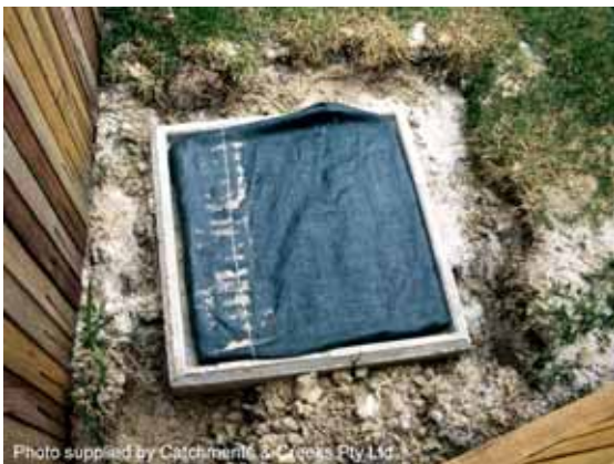
Photo 7 – Fabric wrap drop inlet protection
