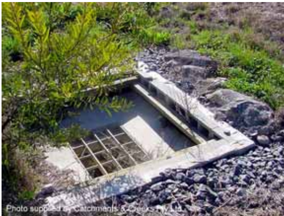
Photo 3 – Block & aggregate system
