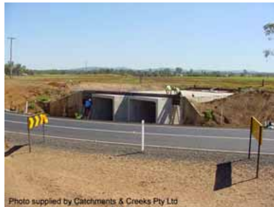
Photo 2 – Culvert inlet
