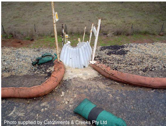
Photo 1 – Batter chute formed from corrugated sheet iron
