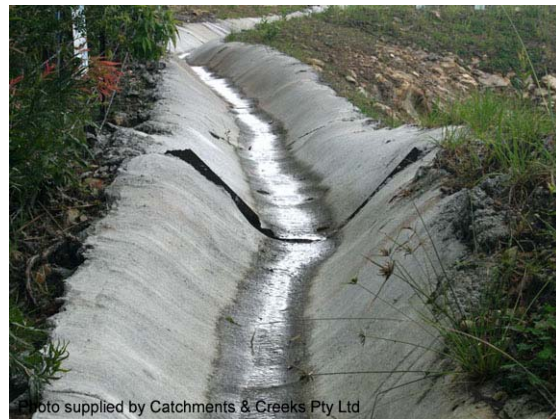
Photo 2 – Concrete lined catch drain
