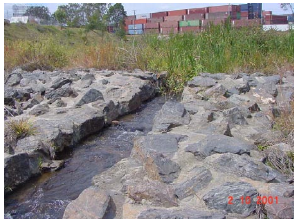
Photo 4 – Low-flow channel through weir crest (note the component of the drop was not damaged due to original concrete grouting)
