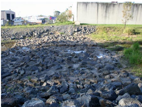
Photo 3 – Repaired structure (grouted rock)
